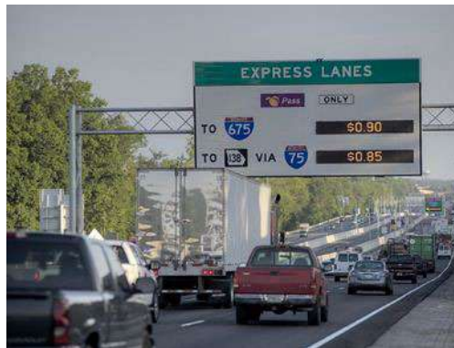
I-75 South Metro Express Lanes
