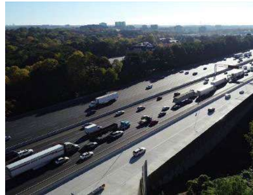
Northwest Corridor Express Lanes
